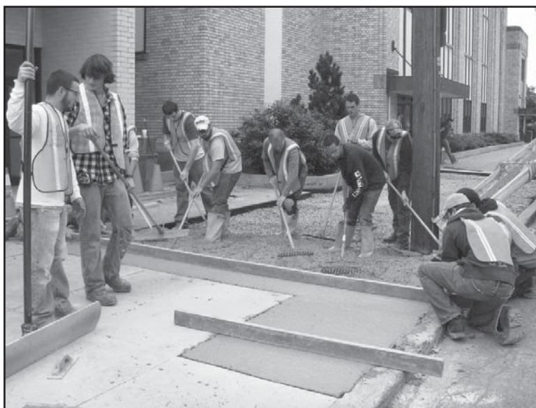
Pennsylvania College of Technology students pouring and finishing sidewalks.
